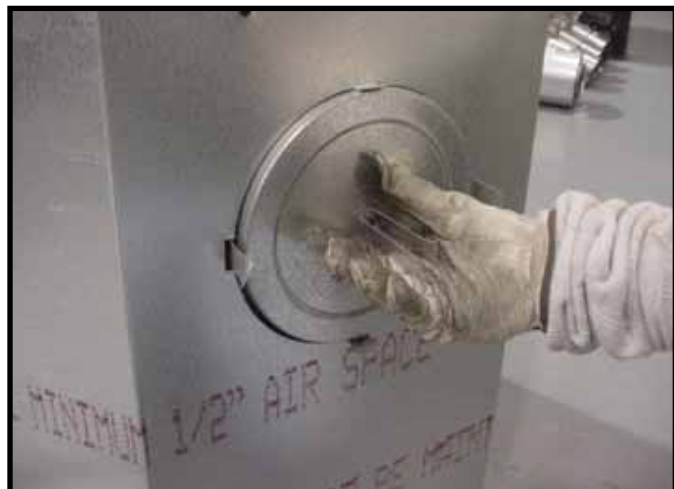
Figure 9.8 Fold the center parts of the retaining band out and use to remove the seal cap.
